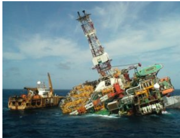
Figure 2.4.: The Petrobras P-36 oil platform sinking.
